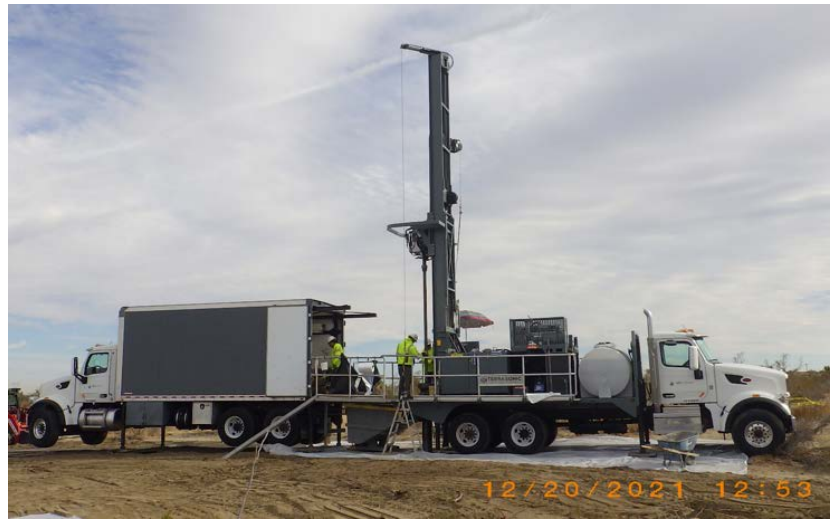
Terrasonic 600 drill rig
