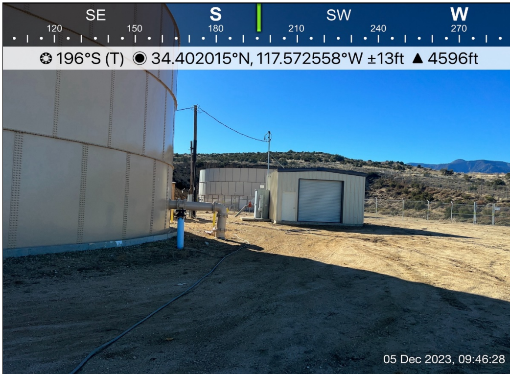
Photo. View of existing Reservoir 6A
