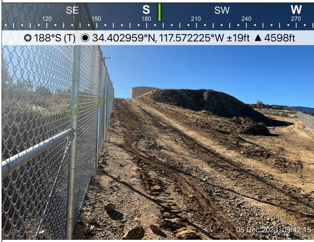
Photo #4 Typical view of south access road.
