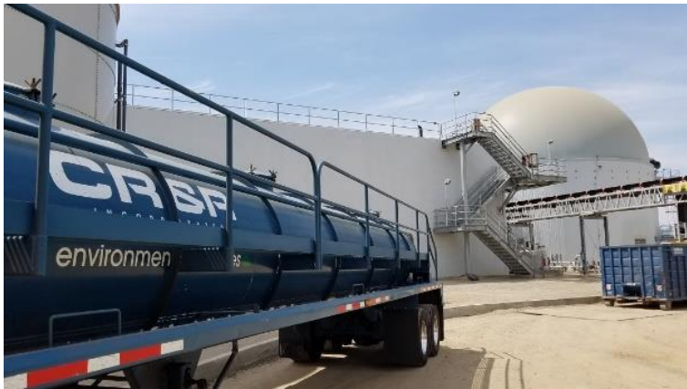
ANAEROBIC DIGESTION FACILITY
